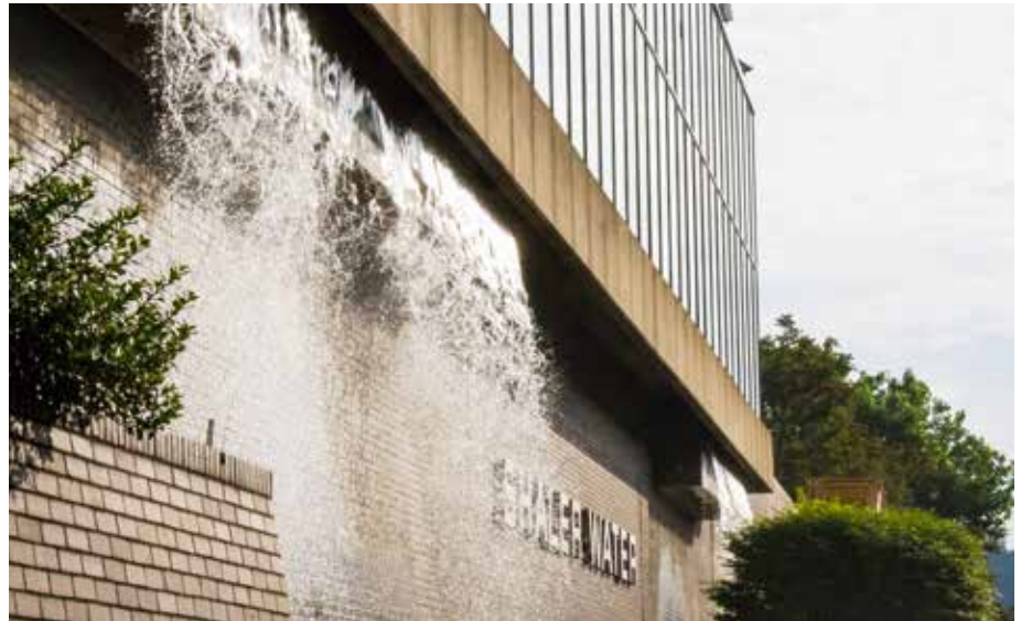
A good example of how engineered, “stand-alone” chemical feed systems can bring results both impressive and sustained can be found at the Hampton Shaler Water Authority.
