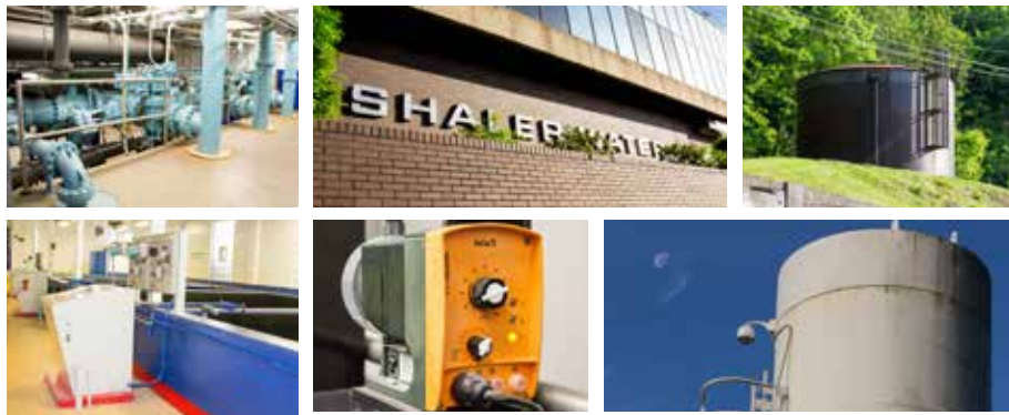
The Shaler Water Treatment Plant draws from 14 wells located along the banks of the Allegheny River. The treatment facility is operated 24/7, has a rated capacity of 9 MGD. The plant is a good example of how incorporating engineered, “stand-alone” systems can bring results both impressive and sustained.
