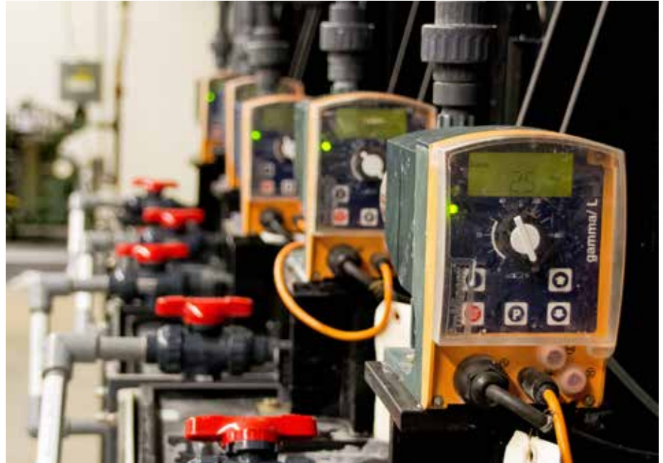
Gamma/L calibrateable pumps are integral to HSWA’s chemical feed skids. The microprocessor-controlled solenoid metering pumps provide for electronic variable speed control, and a special bleed valve integral to its liquid end minimizes potential for off-gassing issues.
