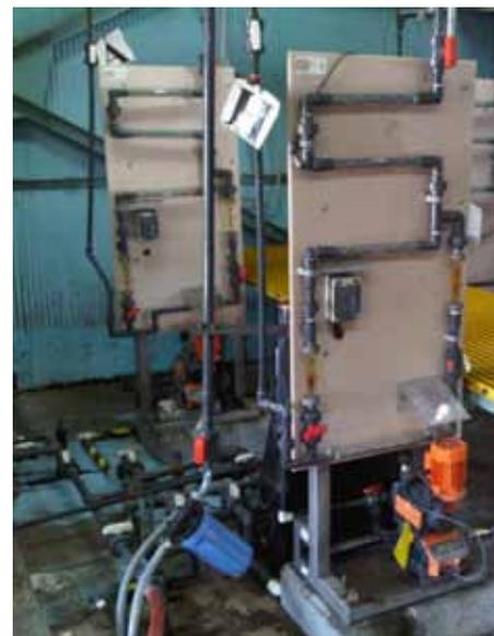
2002 Polymer Make-down system utilizing ProMinent Sigma pumps and static mixers.
