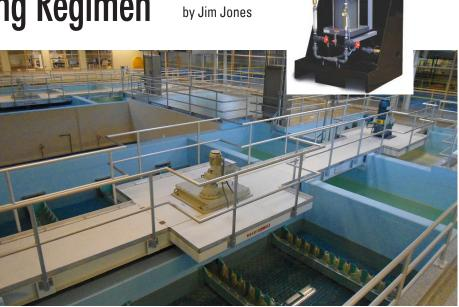
Improved polymer activation and feed at Mankato's Water Treatment Plant, through the addition of a ProMix-S polymer blending and delivery system *(inset photo)*, has brought improved solids settling in the plant's softening reactor, especially at higher flows.
