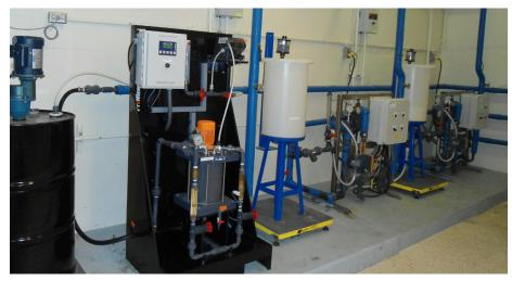
The ProMinent ProMix-S unit provides a multi-zone mixing chamber that delivers a tapered energy profile for hydrating and mixing polymer to a homogeneous and fully activated solution. To the right of it is the plant's former single zone system, requiring day tanks that feed from the 55-gallon supply drum.
