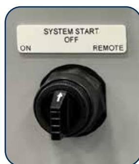
'SYSTEM START' Switch defines where the 'Enable' comes from. (Leave 'OFF' until step 8 below)
