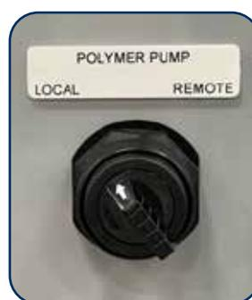
'POLYMER PUMP' Switch defines where the polymer pump 'Speed Control' comes from.
