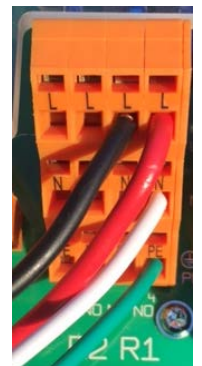
Figure 24 R1 MOV Wiring example
