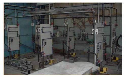
2001 Polymer Make-down utilizing LMI pumps and static mixers. The LMI pumps were replaced in 2002 with ProMinent Sigma 1 Control series pumps; control improved immediately.
