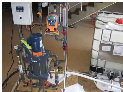
Cake solids are up, now averaging 19%, compared to 14-17% prior to switching to inline polymer preparation and feed.
